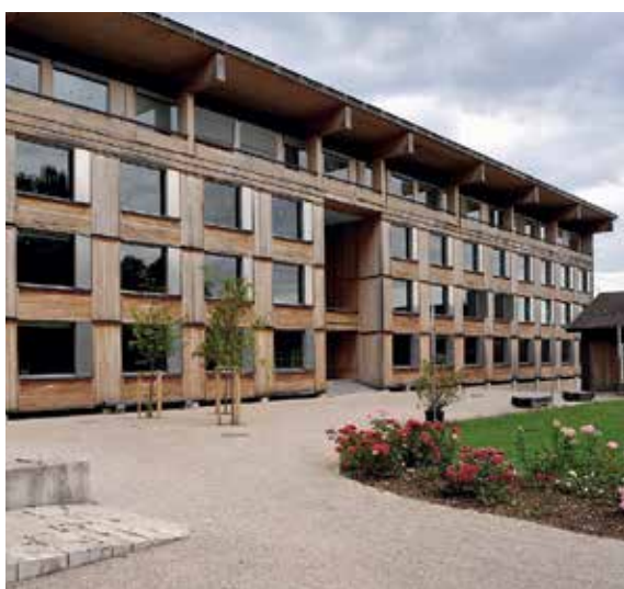
Bern UAS – School of Architecture, Wood and Civil Engineering in Biel.
